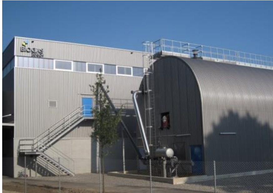
Figure 14: Thermophilic biowaste reactor of Biogas Zürich (© Biogas Zürich)
