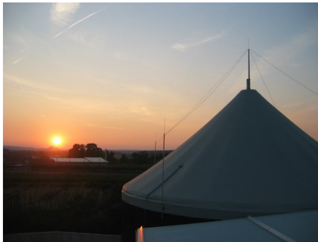
Figure 1: Biogas plant in Strem nearby Güssing
