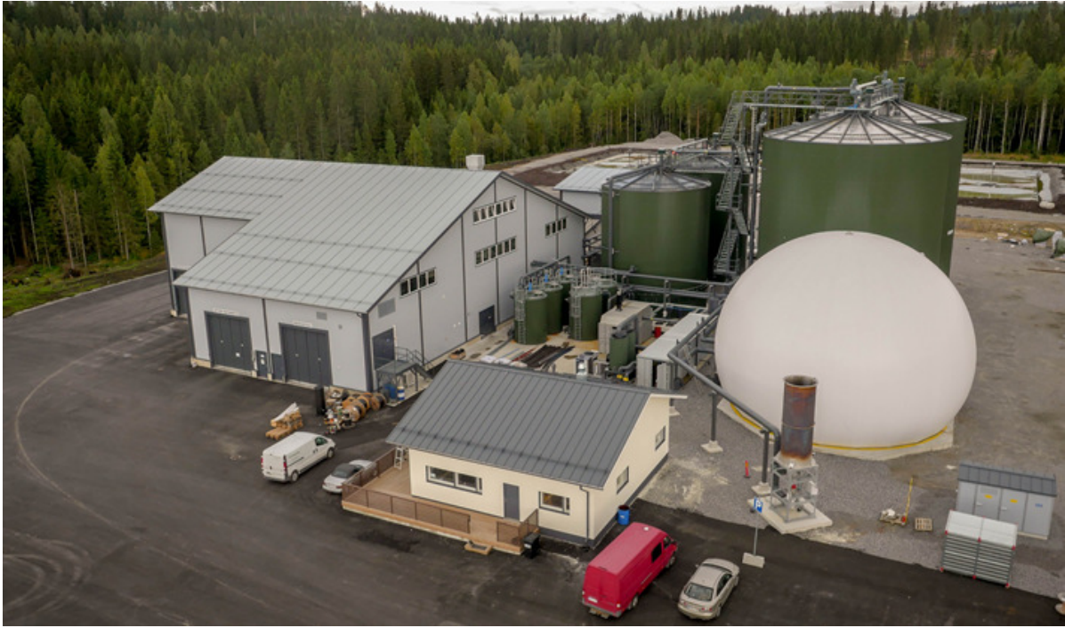
Figure 5: Biogas plant in starting phase in Kuopio. The plant has capacity of 60,000 tonne/year of sewage sludge, source separated biowaste, biowaste from grocery stores and supermarkets, and food industry wastes. Biogas production is about 34 GWh / year, and the biogas is delivered through a 5 km pipeline to Kuopio Energy that produces heat and electricity for Kuopio city.
