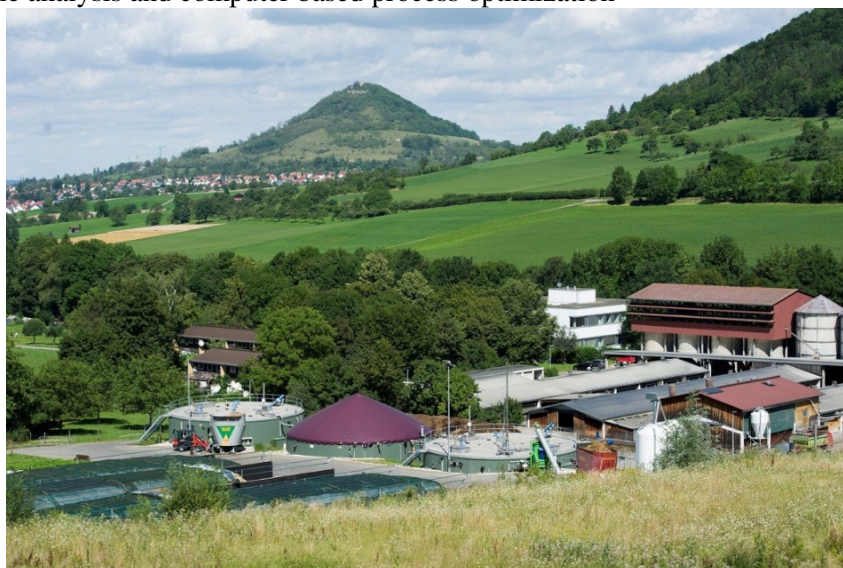
Figure 7: Experimental biogas plant of Hohenheim University
