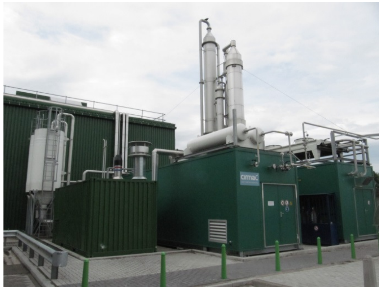
Figure 15: The biogas plant owned by De Meerlanden Rijsenhout that is producing green gas, CO 2 , heat, compost and water
