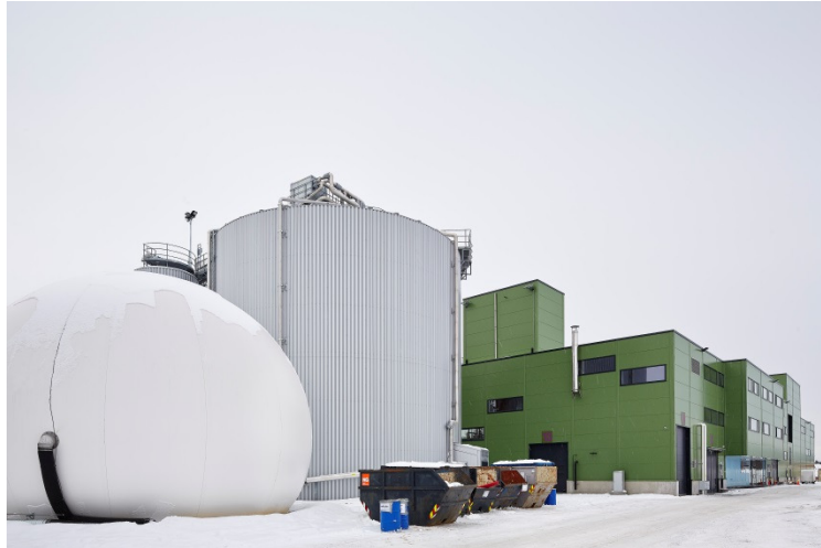
Figure 9: Romerike Biogas plant was operative by the end of 2012. The plant recovers biogas and fertilizer from source separated food waste from the households and businesses in Oslo. (Photo: Oslo Waste-to-Energy Agency)
