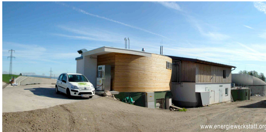
Figure 2: The biogas plant Graskraft Reitbach.
